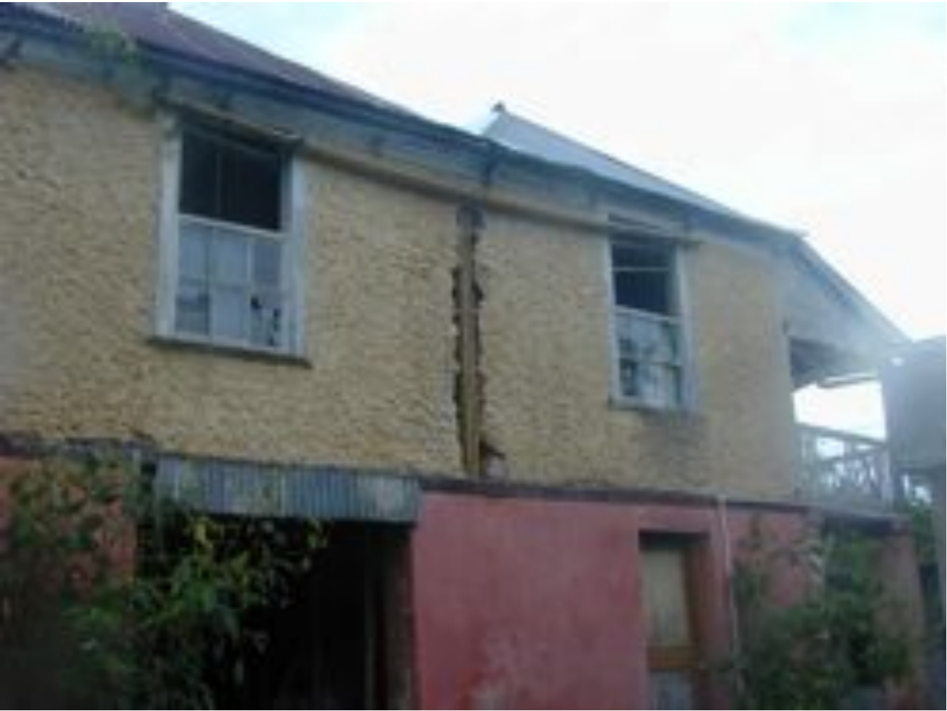
Figure 5 Photo of east side of house showing new post and clamps.
