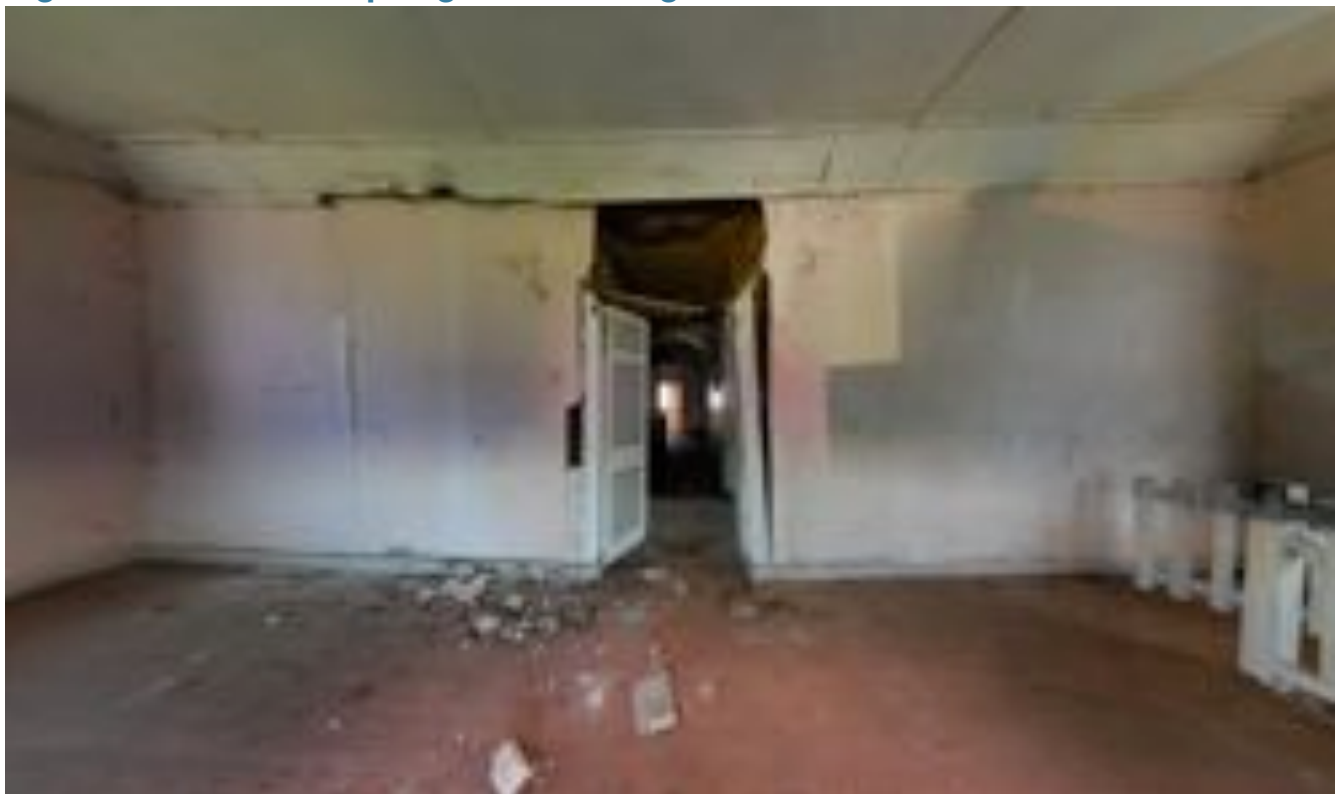
Figure 3 View of collapsing wall in Living Room before intervention
