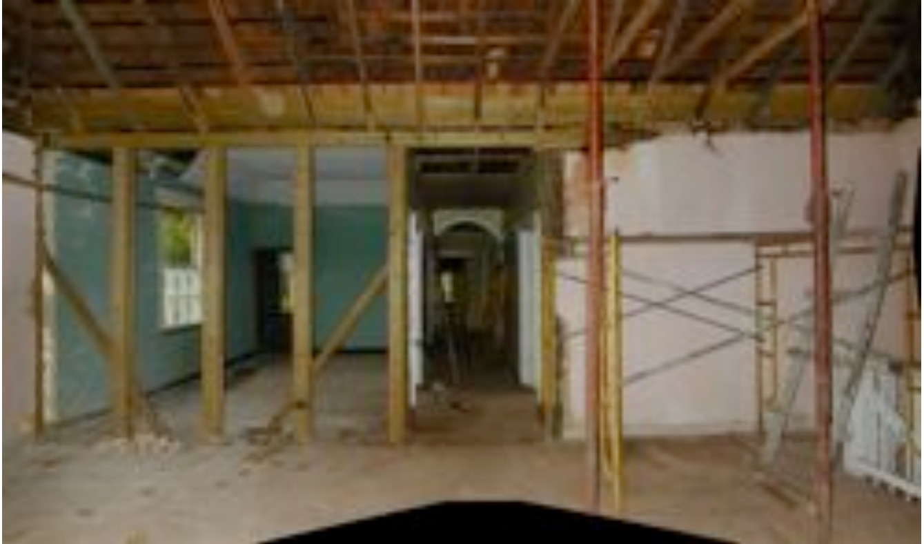
Figure 3 View of collapsing wall in Living Room before intervention
